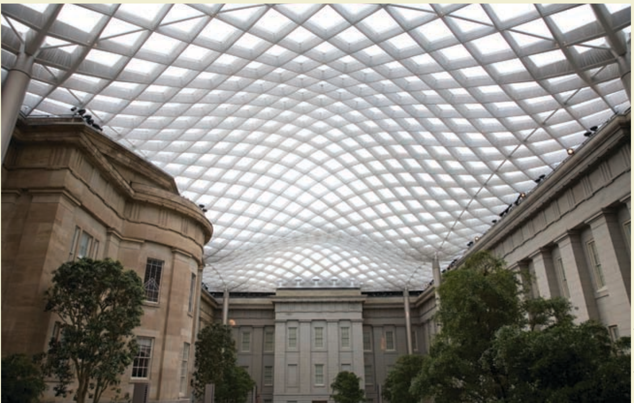
The steel canopy comprises 862 1.6-inch thick double-glazed glass panels. No two are shaped the same. The space includes a variety of plants, two sixteen-foot-tall ficus trees, and sixteen black olive trees.
